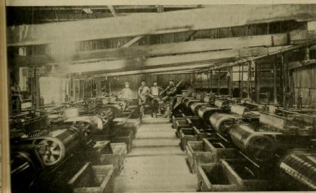
INTERIOR OF GWIN MILL CONCENTRATING PLANT.
